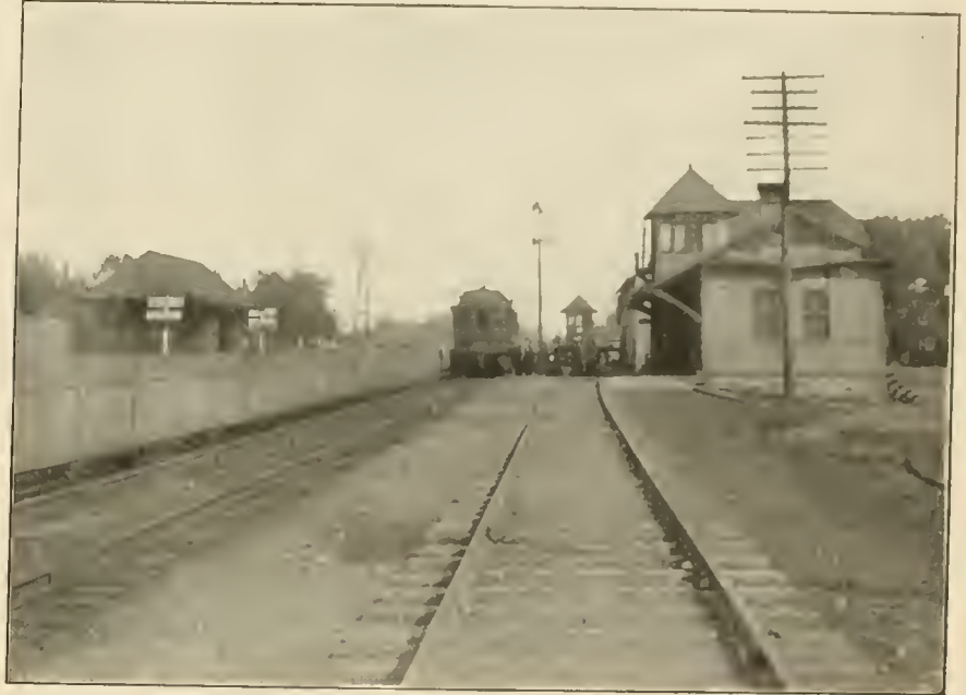
ELECTRIC EQUIPMENT ON THE WEST SHORE RAILROAD.
